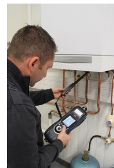
Ambient CO checking
